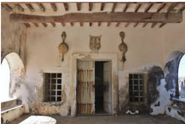
Chapel of Nossa Senhora do Baluarte (facade)
