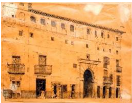
Facade of the palace of Cetti Meriem or house of the Infantes
