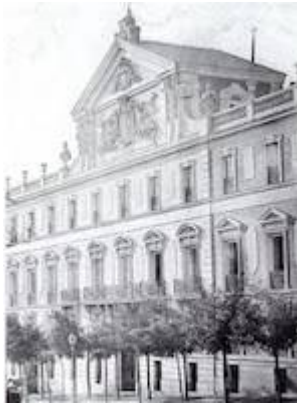
Medinali's main door palace
