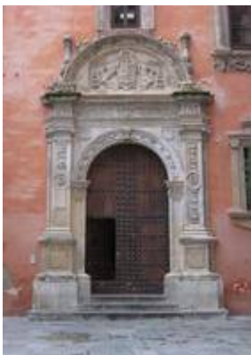
Facade of the Colegio Real (University of Granada). Picture by Juan Ruiz Jiménez
