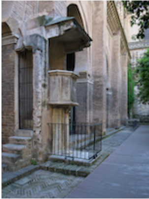
Pulpit of the Orange Tree Courtyard
