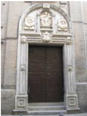
Facade of the hospital of the Corpus Christi. Picture by Juan Ruiz Jiménez
