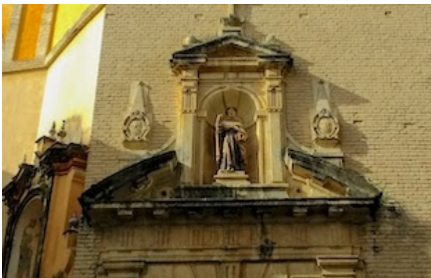
College of San Alberto. Foundation and library.
