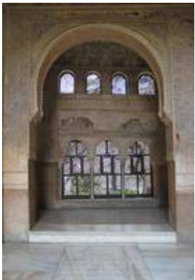
Chapel of the convent of San Francisco de la Alhambra (inside). Picture by Juan Ruiz Jiménez
