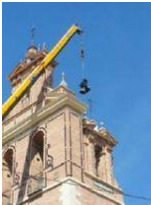
Placing a bell in the belfry of the church of San Juan de la Palma
