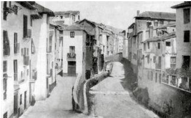
Bridge of the Gallinería or the San Francisco (1865)
