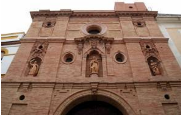
Church of Buen Suceso. Facade. Picture by José Becerra
