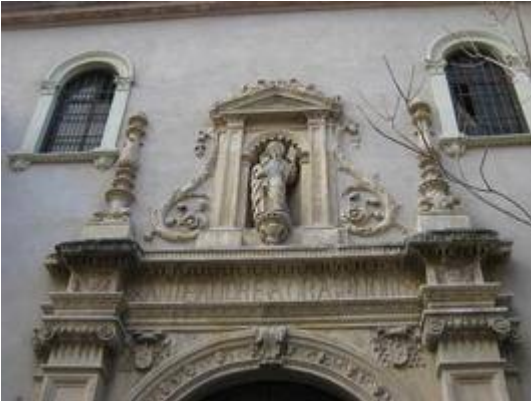
Detail of the facade of the church of San Andrés. Picture by Juan Ruiz Jiménez
