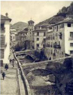
Cabrera and Espinosa bridges
