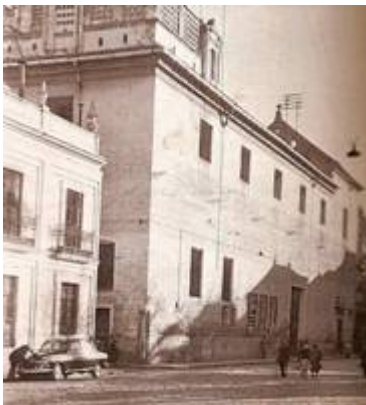
Convent of la Asunción (demolish)
