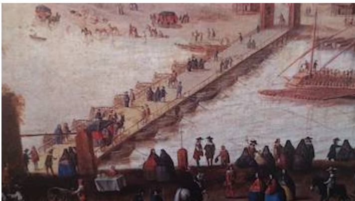
Bridge of Las Barcas (16th. century)
