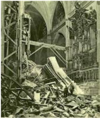
Sinking of Seville Cathedral. Picture by Emilio Beauchy (1888)
